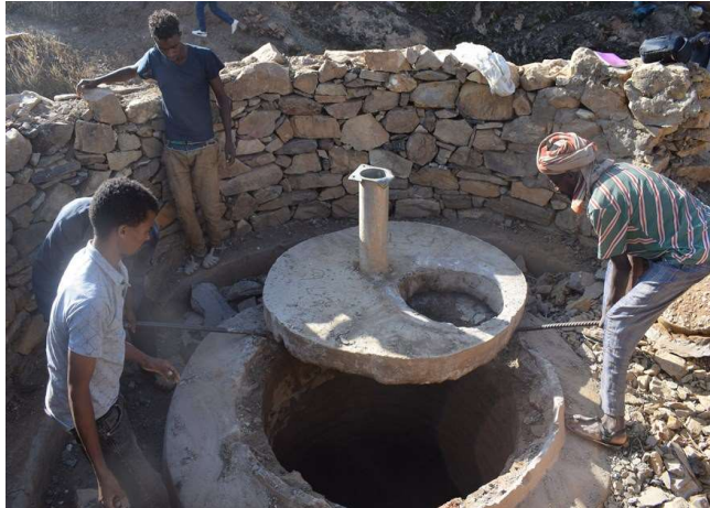
REST workers and villagers repairing the damaged well at Endaba Giray village, Debre Genet district, Tigray
